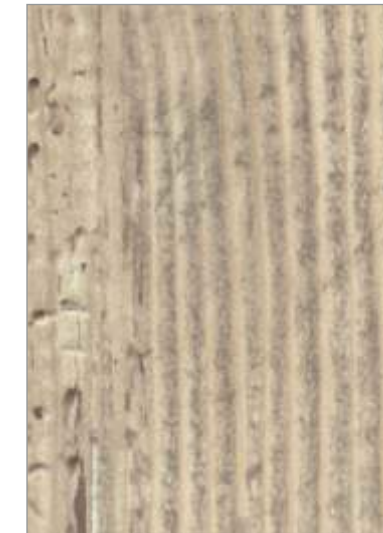
LL 44877 CRACKED WOOD
